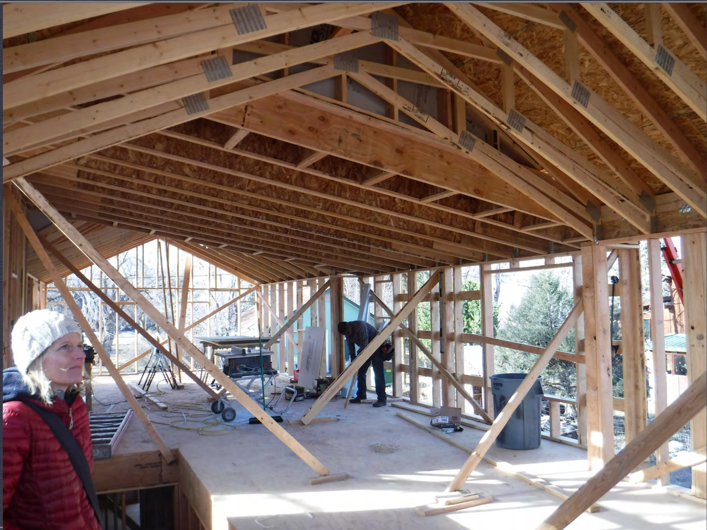
MAR 26 - UPPER LEVEL TRUSS INSTALLATION
