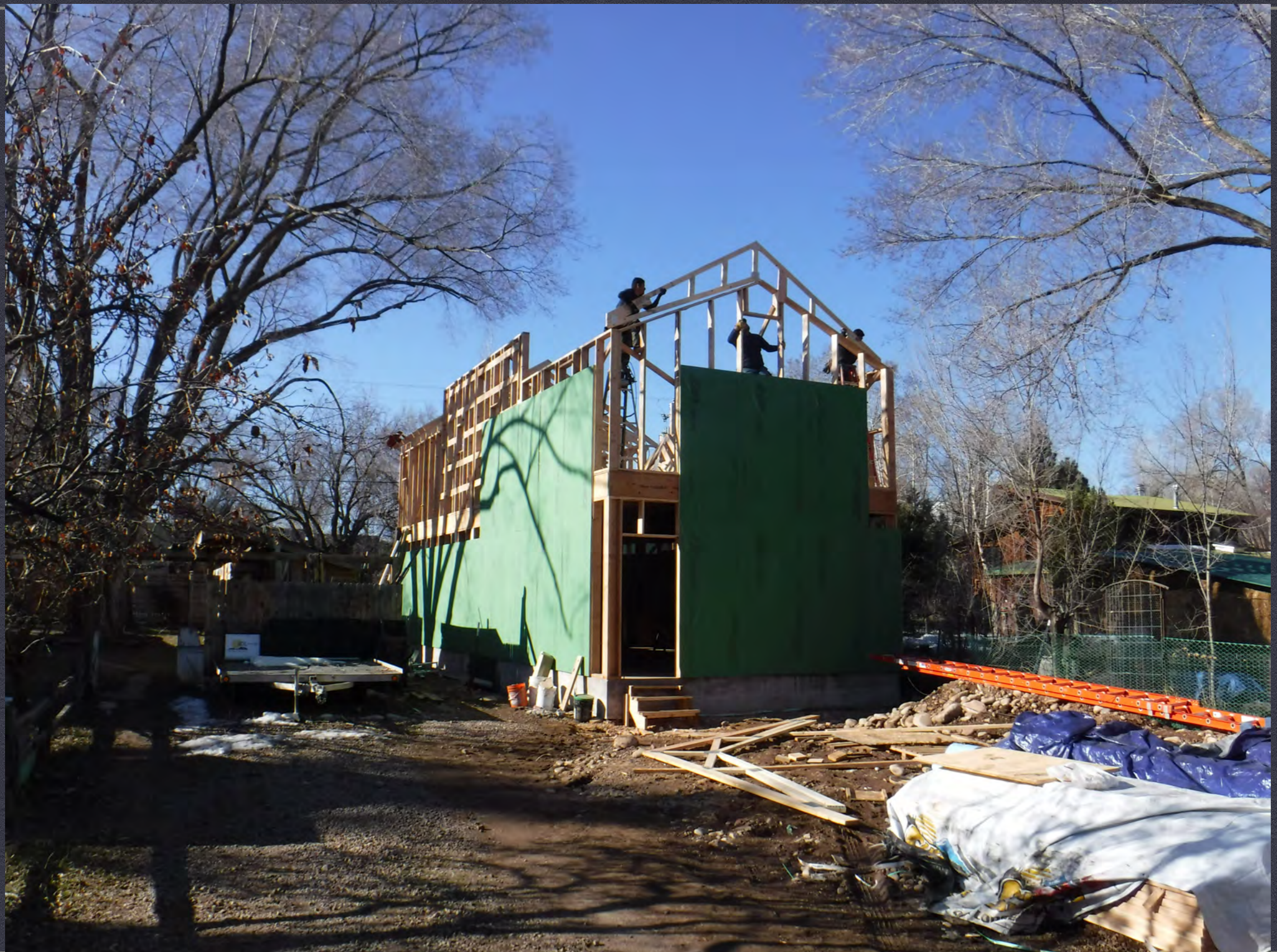
MAR 19 - UPPER LEVEL WALL FRAMING
