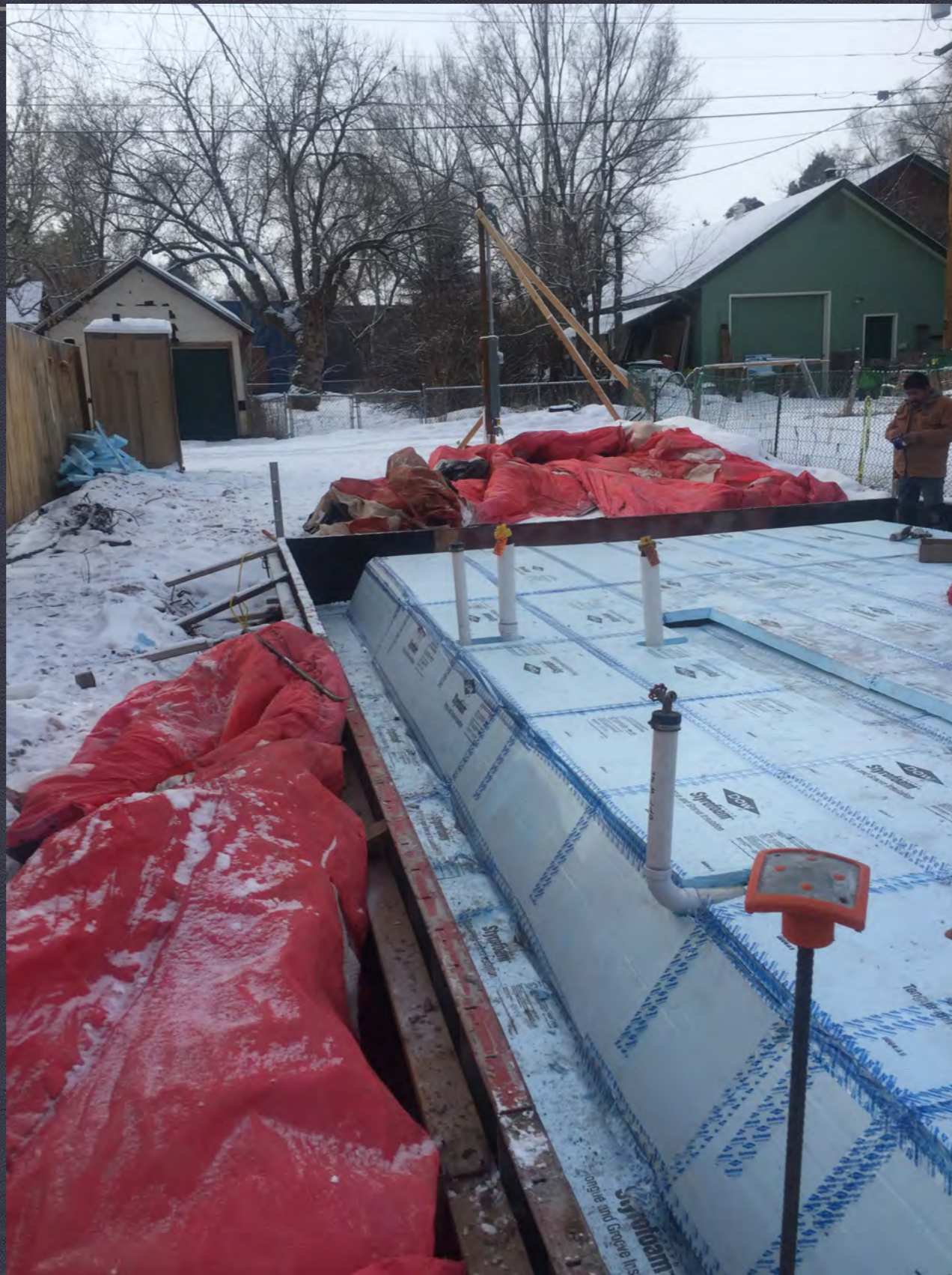
FEB 19 - SLAB PREP
